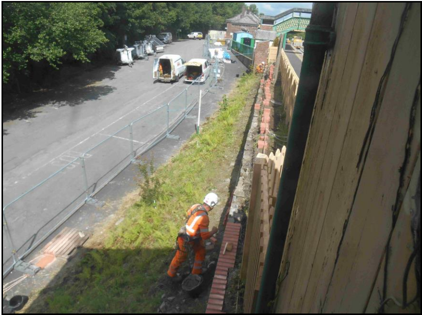
Retaining wall gets new brickwork top.
