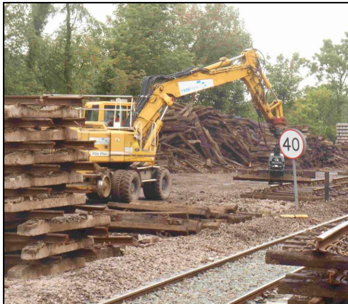
Sorting 11 miles of old track for recycling at Westbury.
