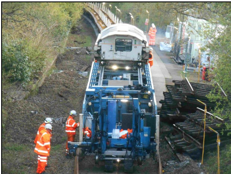
NTCM pauses for maintenance before proceeding under Sampford Courtenay Bridge.
