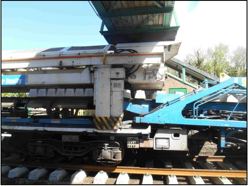
New Track Construction machine straddle carrier under footbridge.
