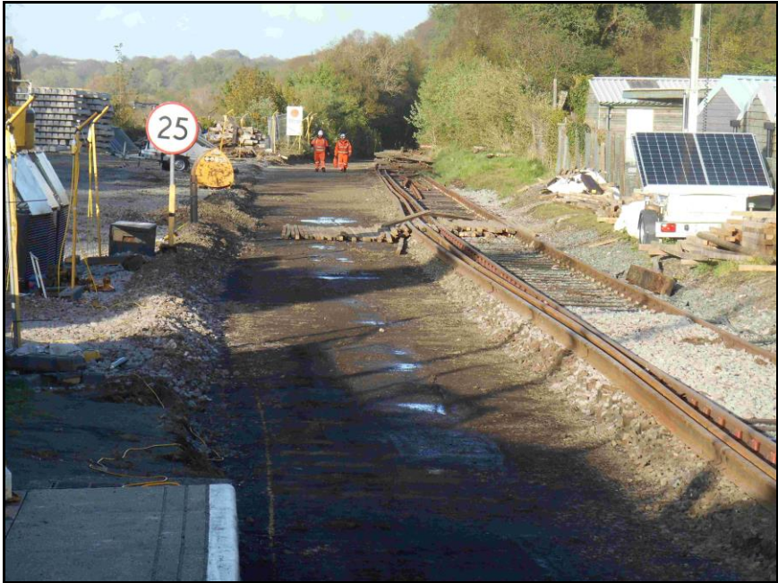
No upside track.
