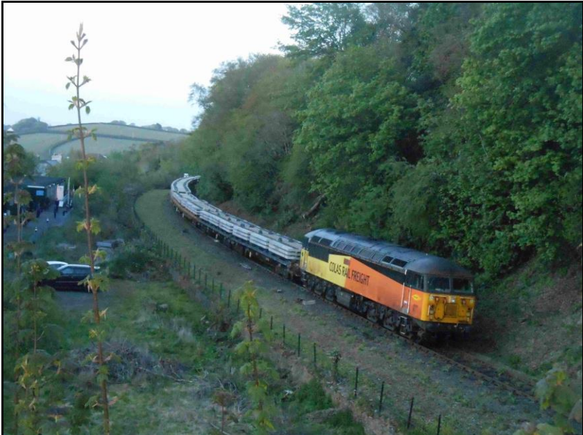
56302 'Peco' with a train of concrete sleepers.
